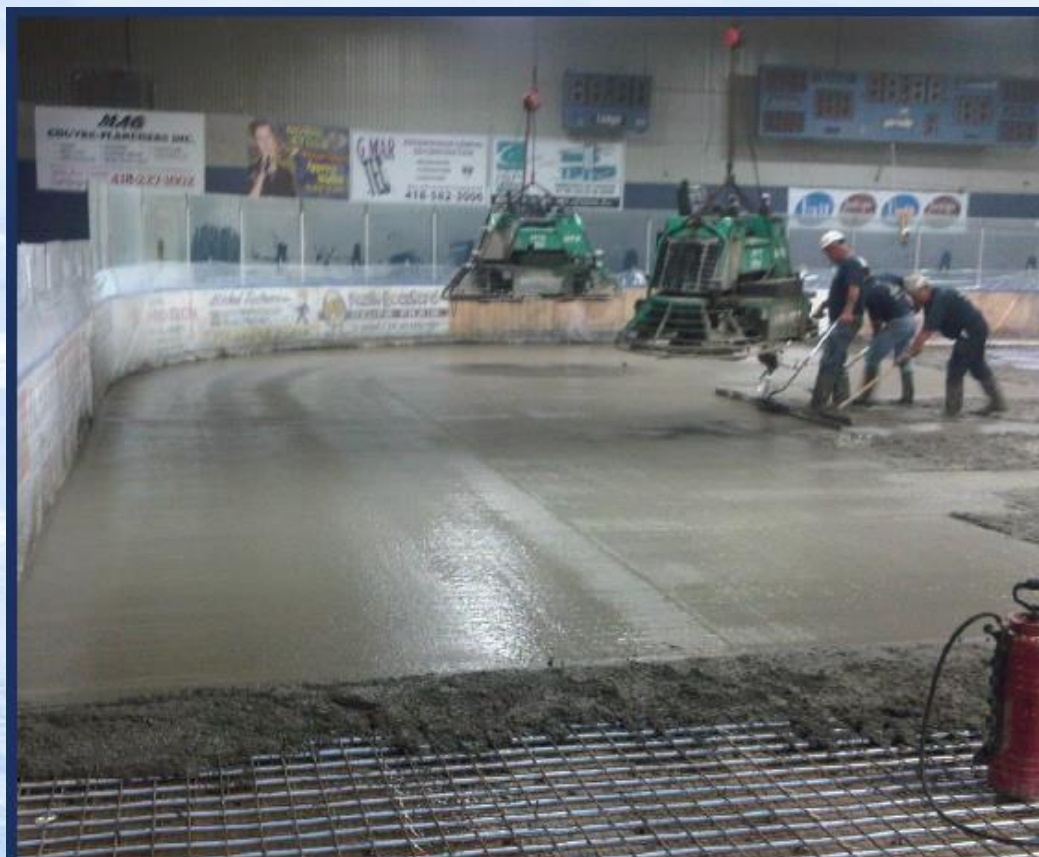
Photo 1: Concrete poured over new copper tube network.
