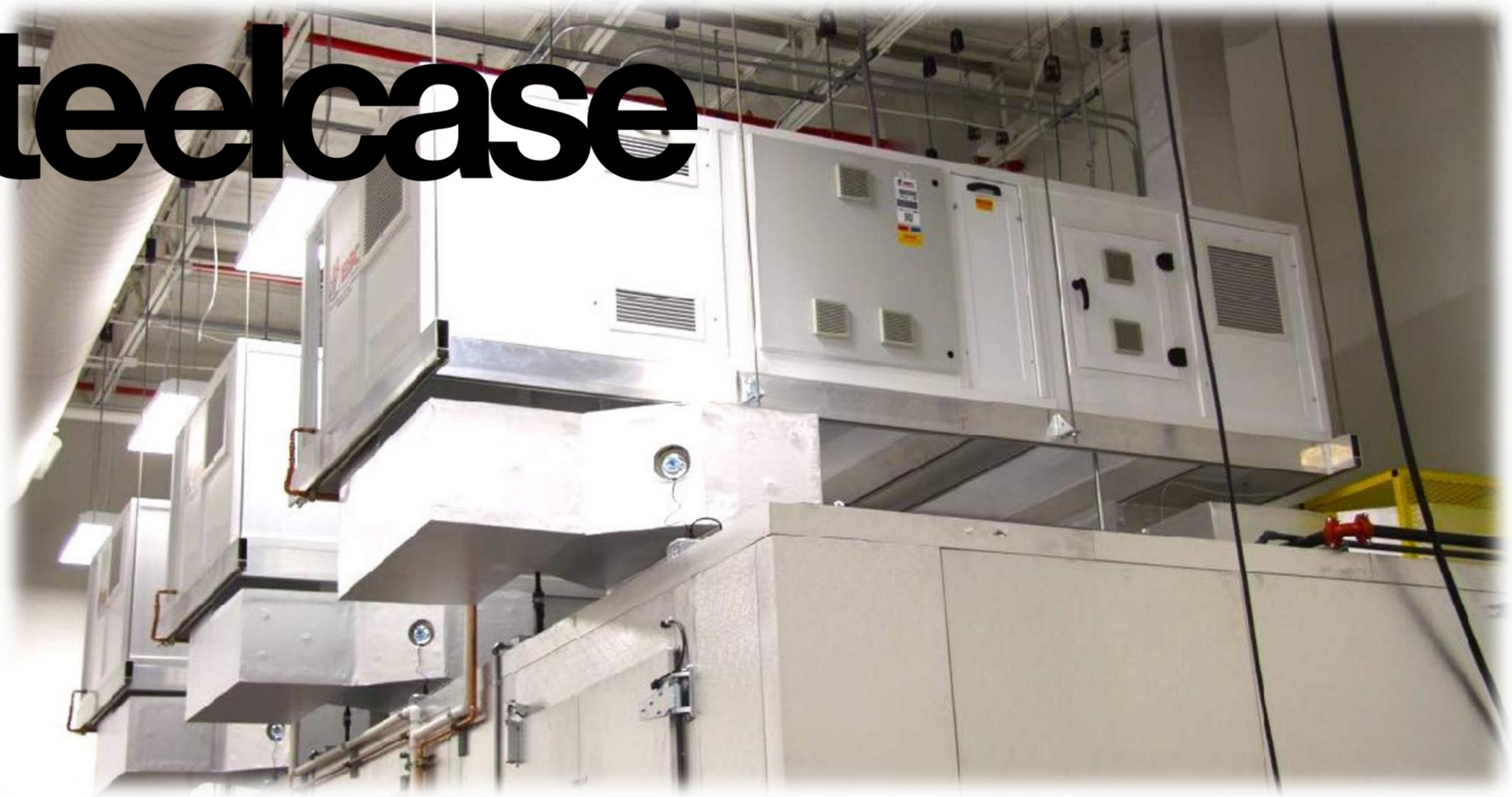
**DESIGN CHALLENGE:** Client originally specified 3 different test chambers, one for dry/hot, one for humid hot & cold, and one conventional office temperature / humidity.
