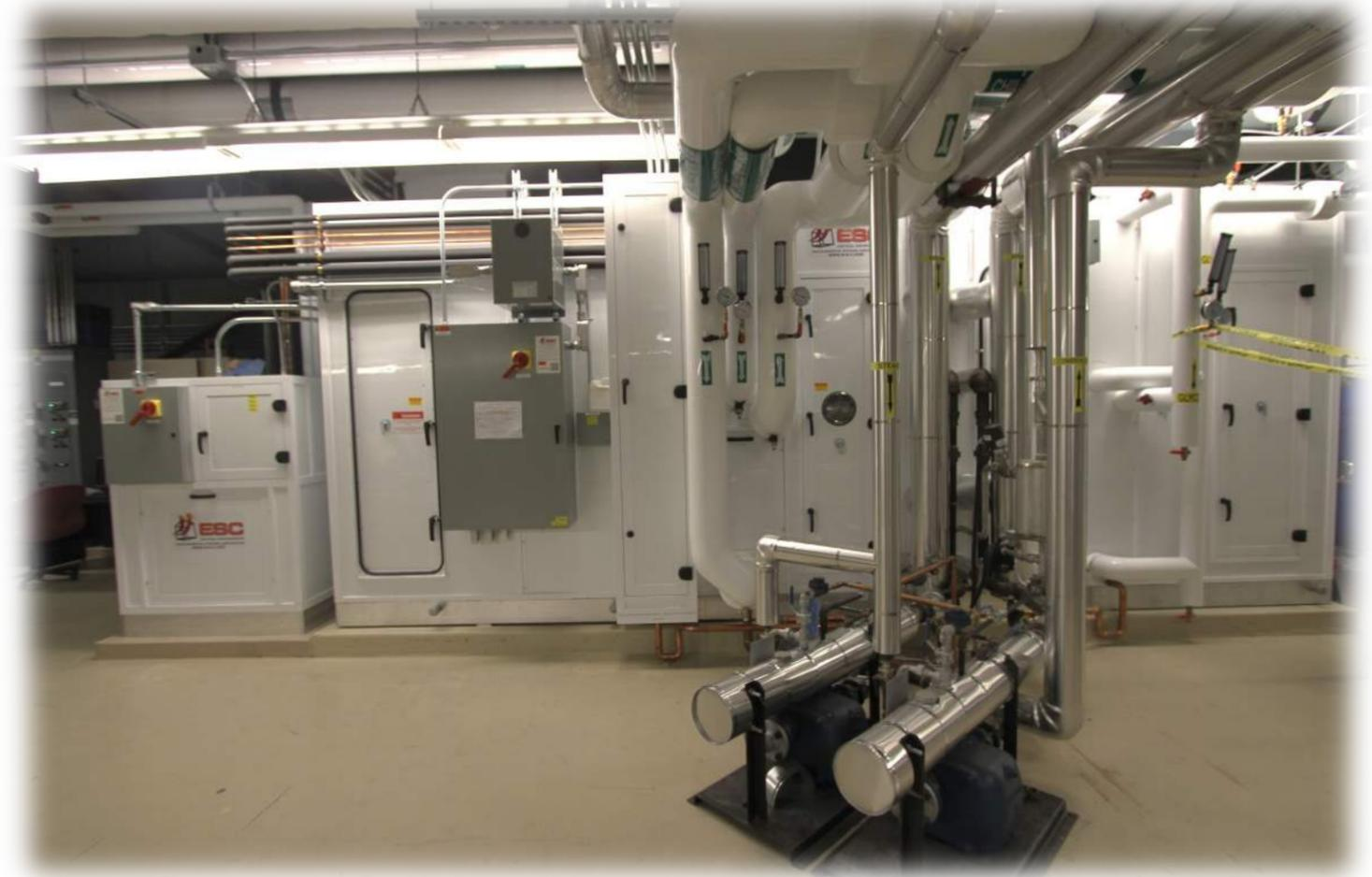
**DESIGN CHALLENGE:** 20,000 CFM Recirculating AHU, becoming a 30,000 CFM MUA.
