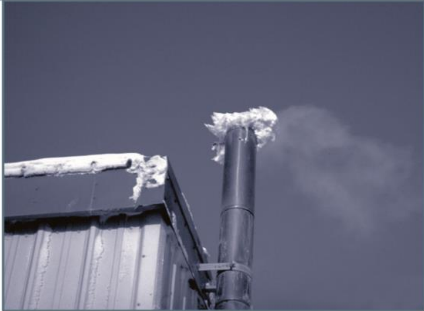
FIGURE 5: FROZEN FLUE UNINSULATED FLUE Richard Armstrong
