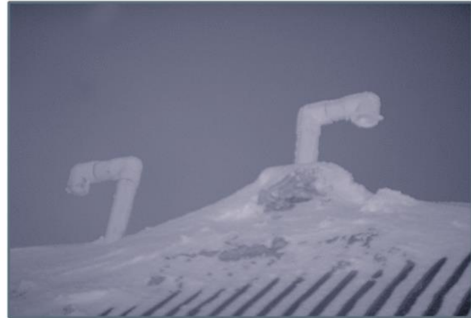
FIGURE 6: PULSE FURNACE AIR INTAKE/EXHAUST FREEZING OF INLETS AND EXHAUST PIPES Richard Armstrong
